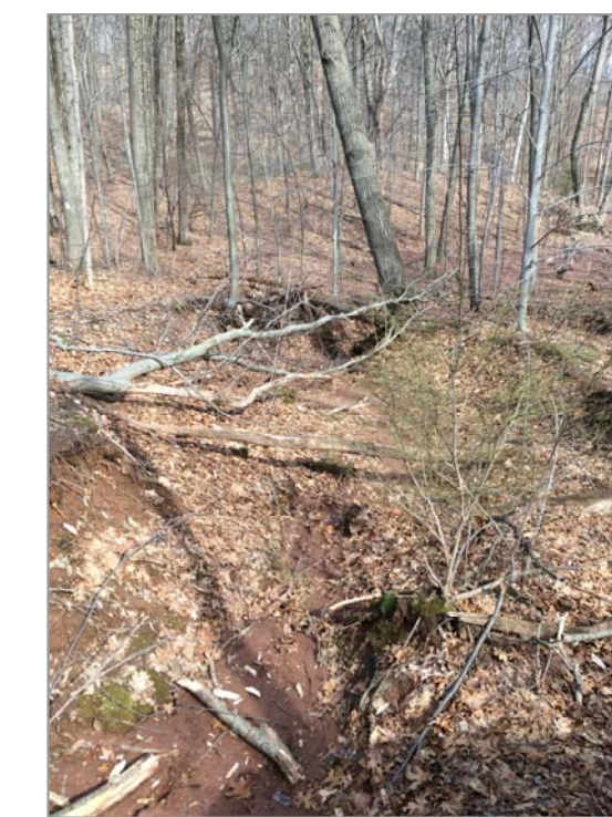
Erosion Creating Ditch 4/15/15 Photo 6
