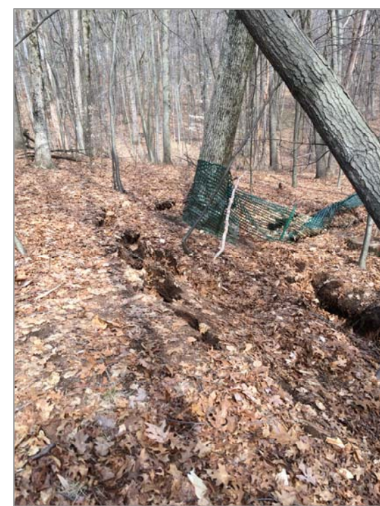
Sloughing at Outlet 4/13/15 Photo 2
