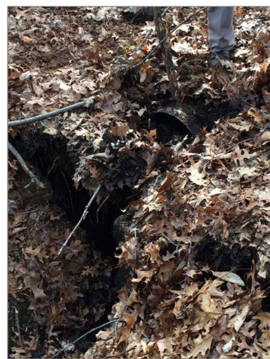
Exist Outlet 4/13/15 Photo 1
